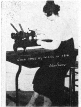
Hand-operated bench lathe for making tungsten coils in 1914 at Westinghouse.
